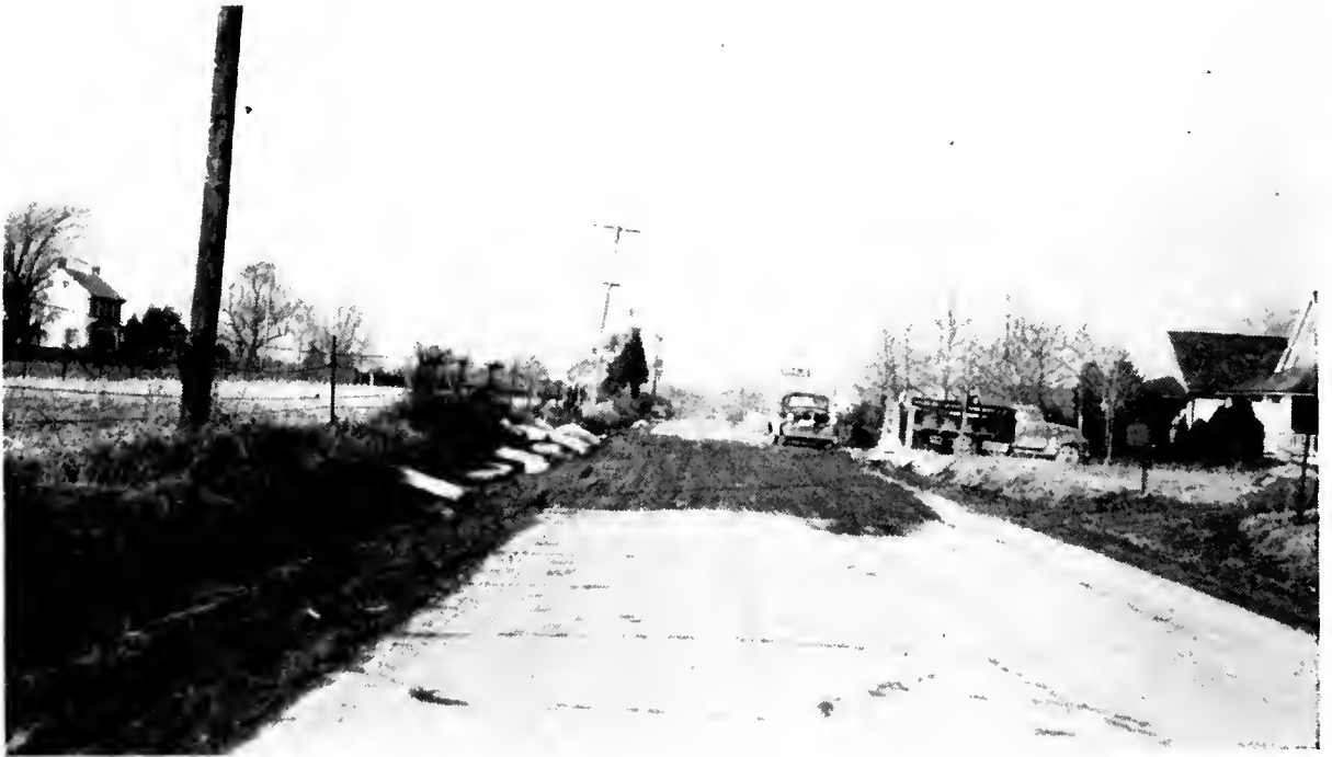
FROST DAMAGE—WINTER 1947-1948—ON U.S. ROUTE 213
